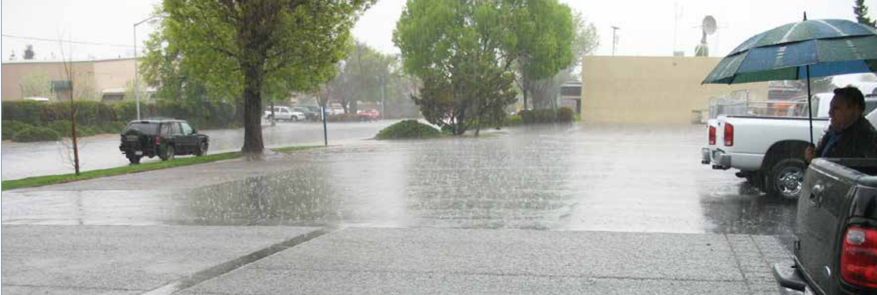
Figure 7.7: Although not as strong as traditional pavement, pervious pavement is suited for low-traffic parking areas.
