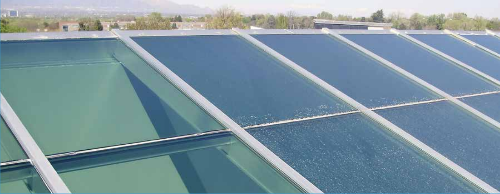
Figure 7.14: Comparison of treated (left) and untreated (right) surfaces demonstrates how titanium dioxide keeps surfaces cleaner.
