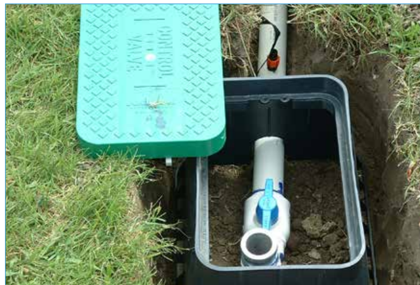
Figure 5.9: System flush valves (in blue) are necessary to periodically remove soil and bacterial contaminants from a dripline. Sediment- or bacteria-containing water is diverted out of the dripline and into the soil. The plastic container housing the valve enables convenient access to it and may limit the area inundated during a flushing cycle.
