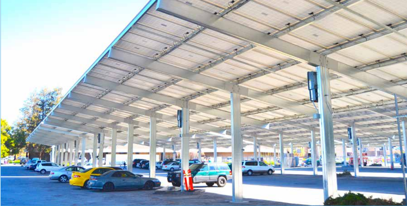
Figure 9.5: A solar shade parking structure provides cover from the sun while generating electricity for other uses.
