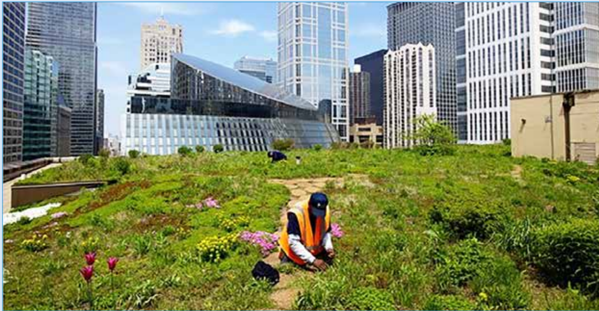
Figure 4.12: Chicago City Hall's semi-intensive green roof provides environmental and cost-saving benefits.
