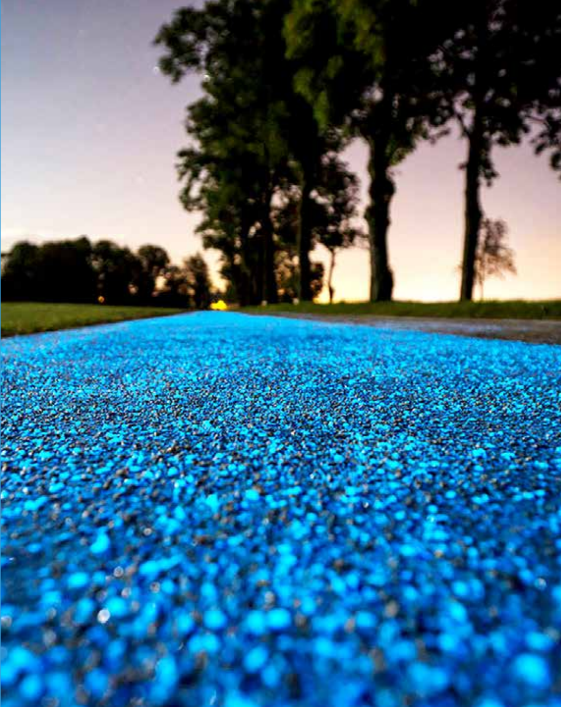
Figure 7.19: Fluorescent pigments can glow up to 12 hours after just 10 minutes of natural light exposure.
