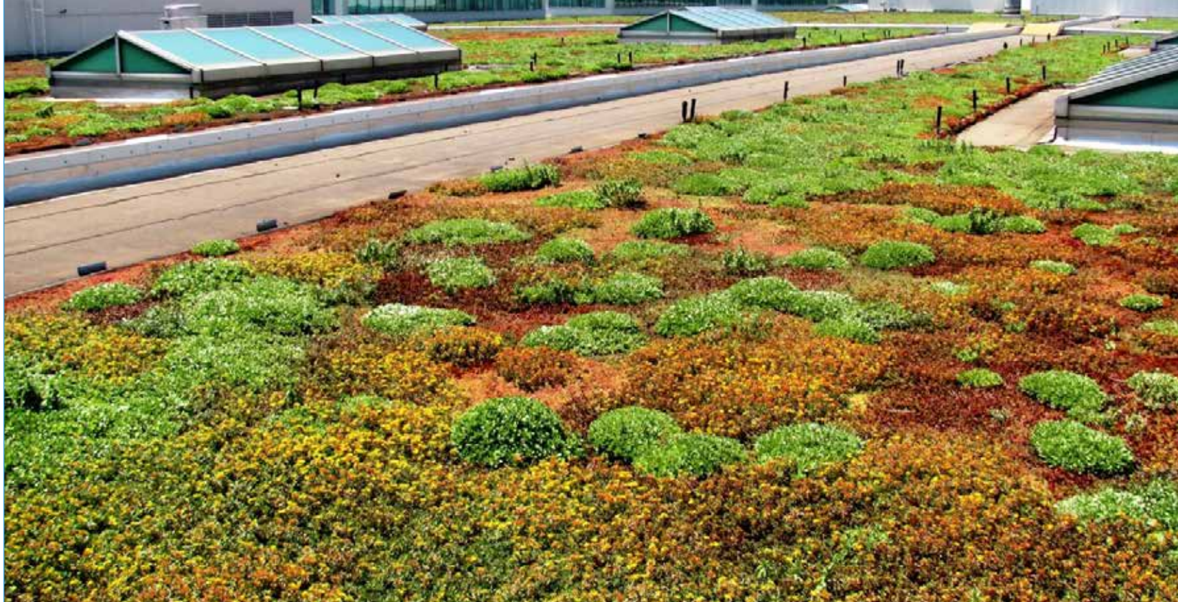
Figure 4:11: Green roofs naturally cool buildings because the vegetation provides shade, absorbs heat, and insulates the building.
