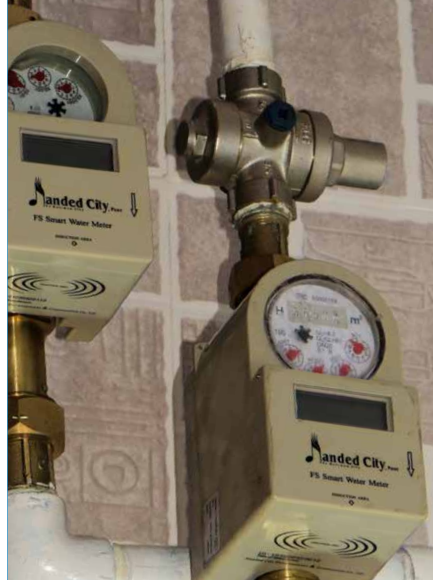
Figure 5.11: With smart water meters, utility staff can access water usage data online and assume real-time control over meter reads and water flows.
