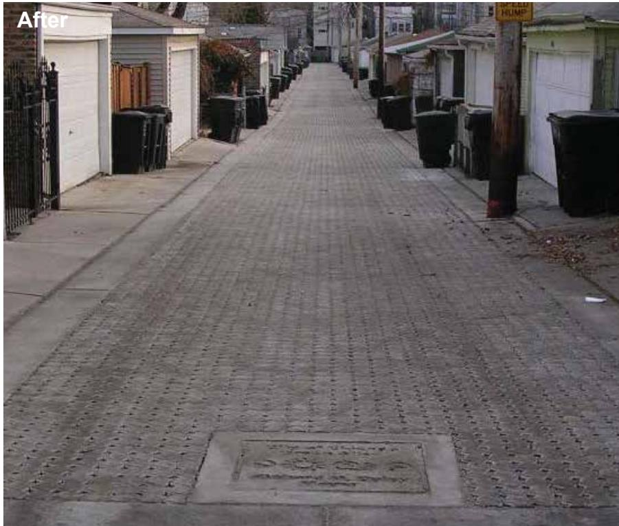
Figure 7: Chicago green alley with permeable pavement that reduces flooding in a cost-effective manner
