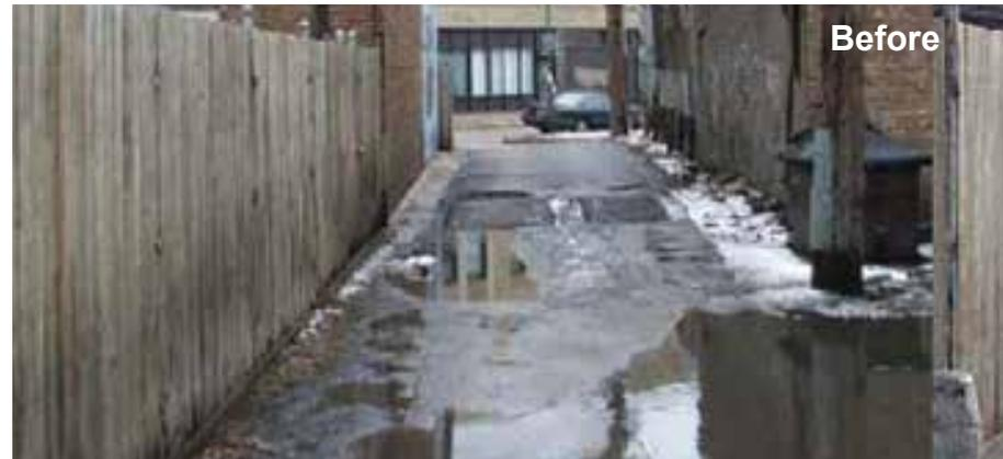
Figure 6: Chicago alley with impermeable pavement and poor drainage before improvements
