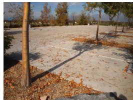
Parking with Infiltration areas
