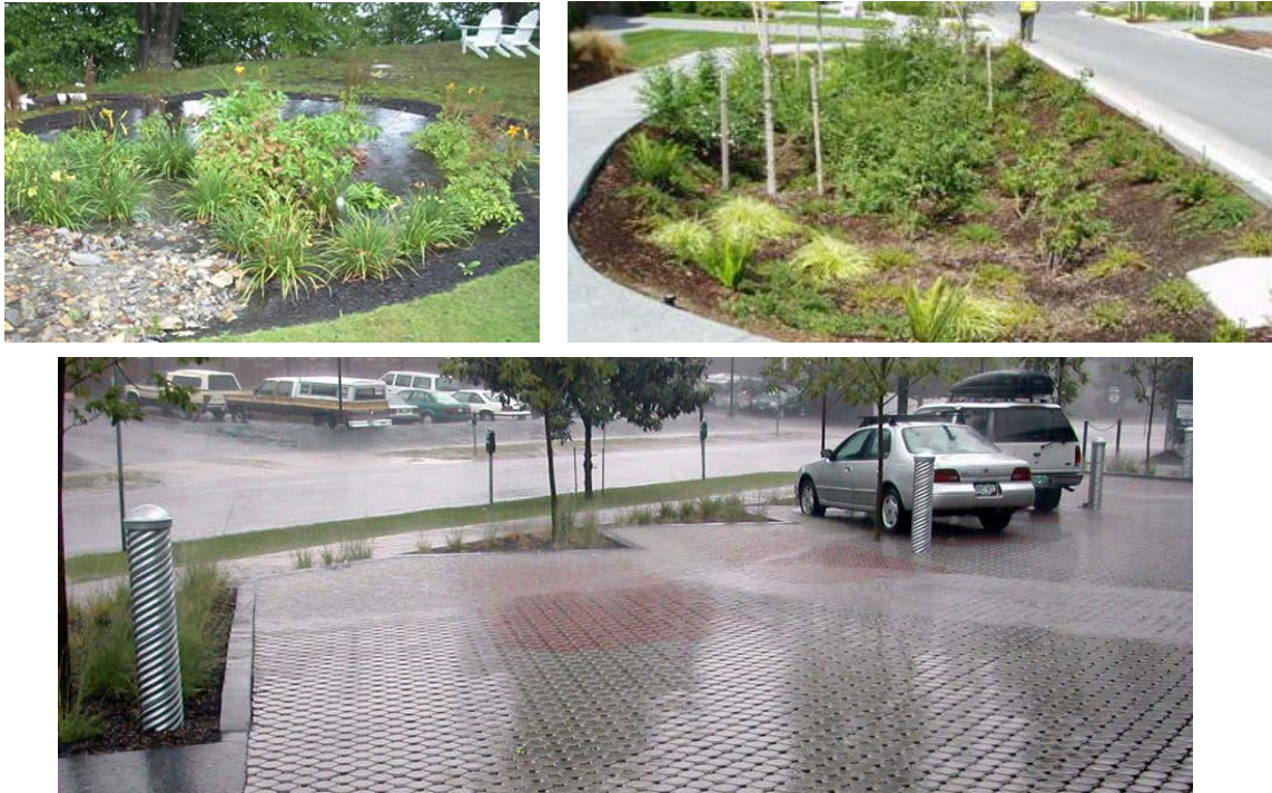
Figure 4-1. Clockwise top left to bottom right: rain gardens, bioswales, and permeable pavement are all green infrastructure solutions that are often incorporated into LID site and building design. Courtesy of U.S. EPA, City of Kirkland, NACTO
