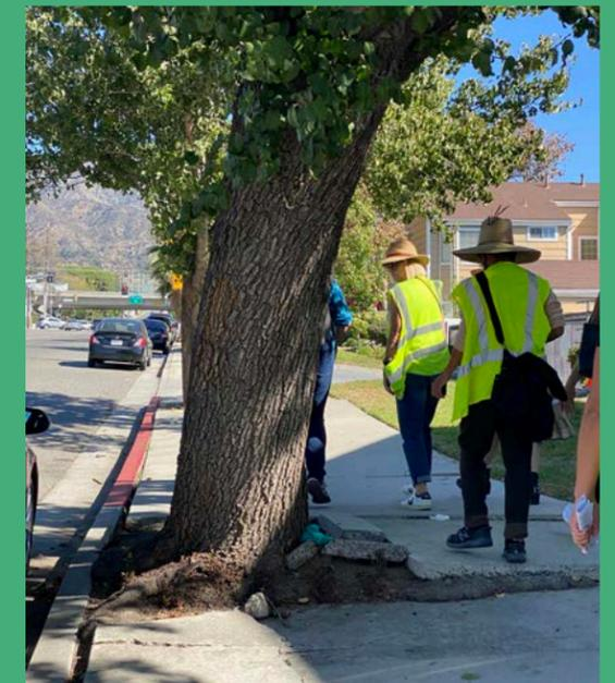
Figure 5. Insufficient tree well size
