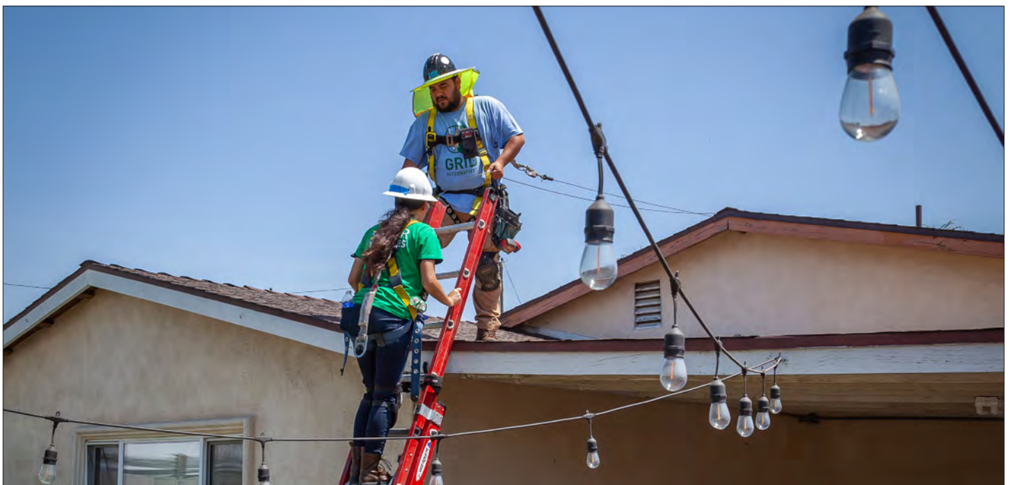
GRID Alternatives installs solar panels in the project area as part of Ontario SHINE. Photo credit: GRID Alternatives
