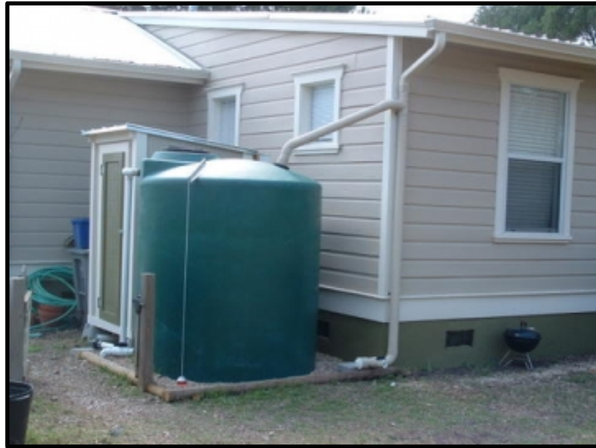
Figure 1. A roof-catchment cistern system
