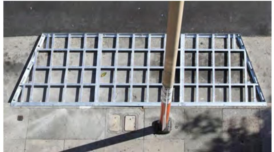
Figure 72. Installed steel sub-structure, "Peace Keeper" parklet, San Francisco, CA.
