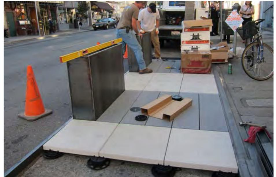
*Figure 81.* Pre-cast concrete pavers during installation, San Francisco, CA.
