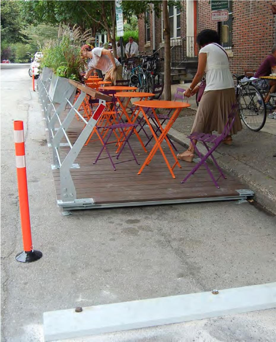
*Figure 46.* Wheel stop and flexible bollard, Philadelphia, PA.
