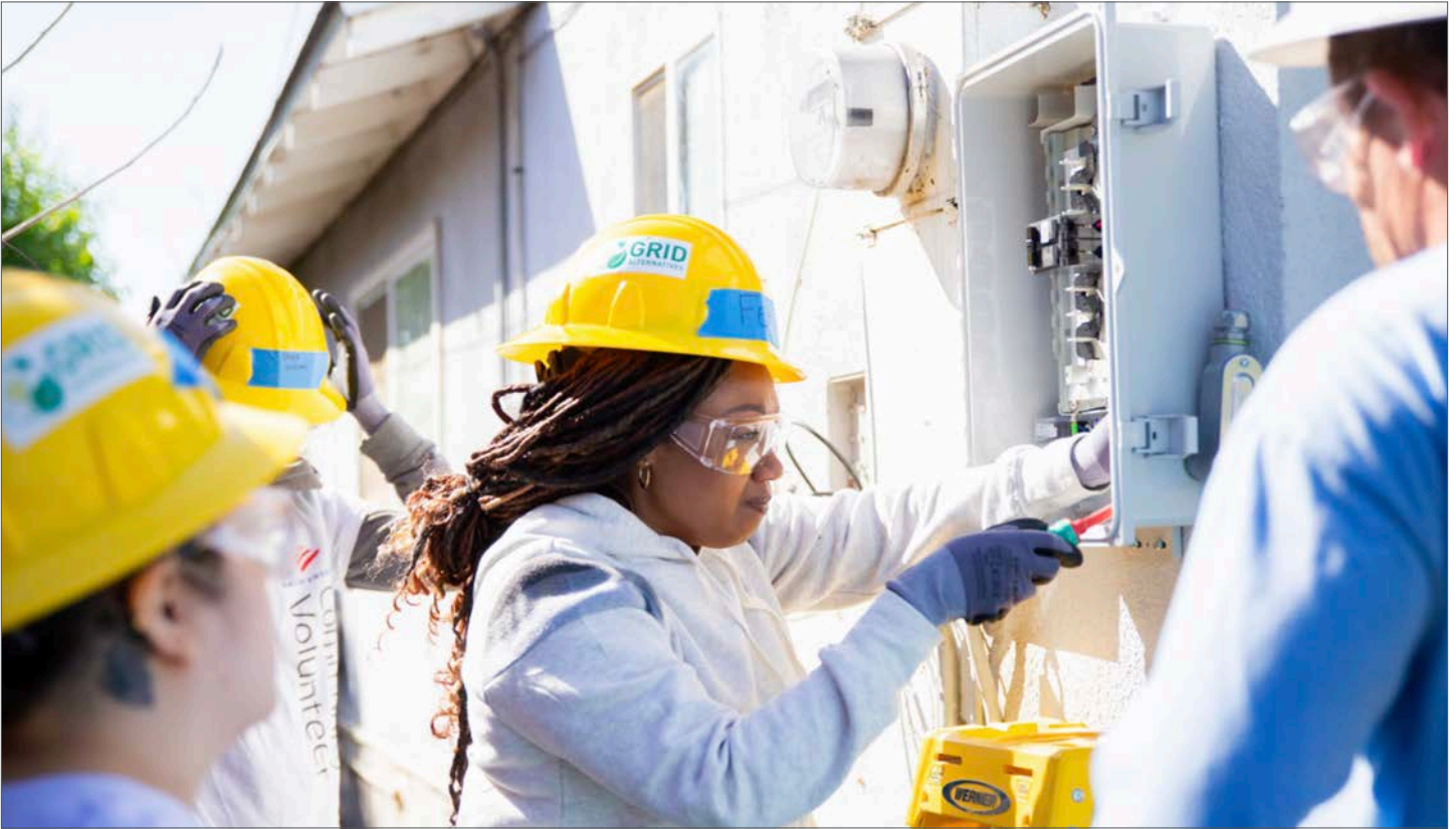
GRID Alternatives trainees upgrading an electrical box to accommodate rooftop solar panels. Photo credit: GRID Alternatives
