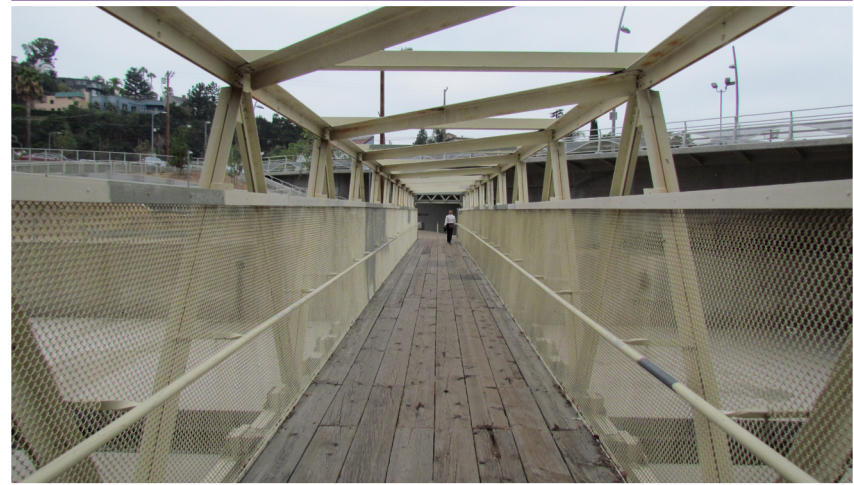
Figure 5 – 35: Colfax Avenue footbridge is a steel Warren through truss structure that incorporates a wood platform. The use of wood is appropriate because pedestrians are low impact.
