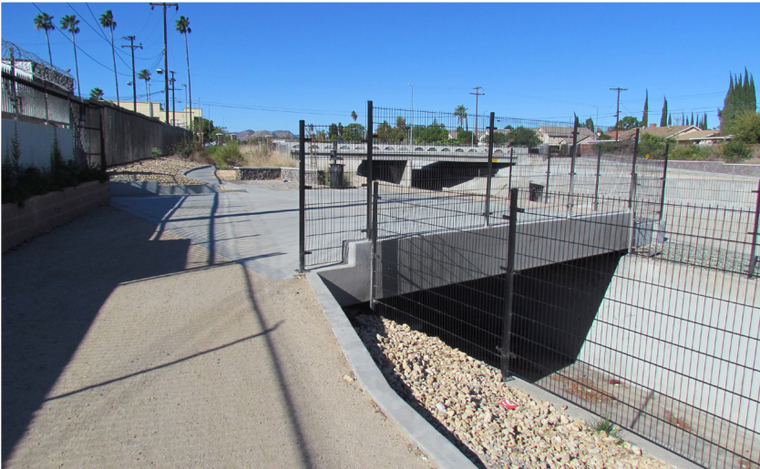
Figure 5 – 1: Simple bridge crossing over a drainage weir enables a continuous pathway connection on the south bank of the Los Angeles River Headwaters project, just south of De Soto Avenue.
