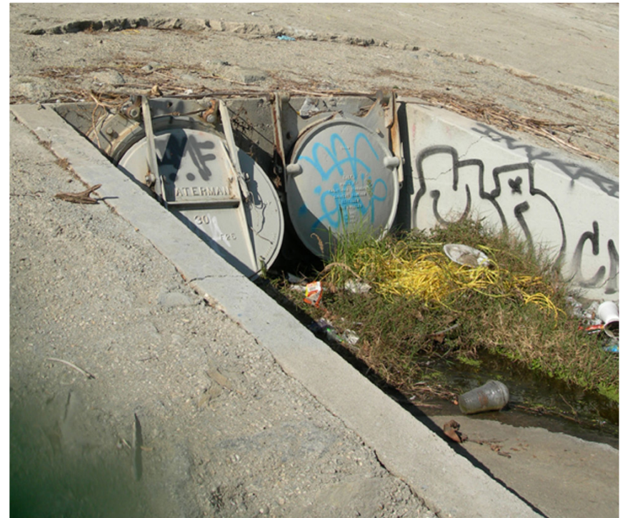
Figure 3 – 11: The site's original storm drains emptying untreated rainwater into the LA River.
