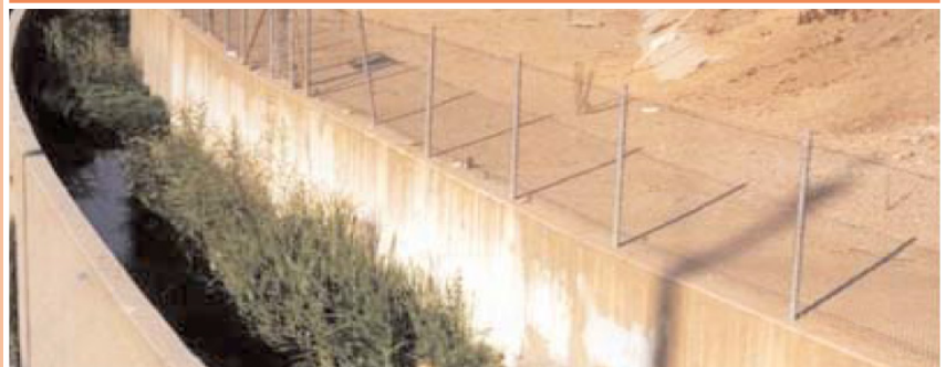
Figure 4 – 16: Weirs, dams that divert or regulate water flow, need periodic cleaning to remove plants and debris.
