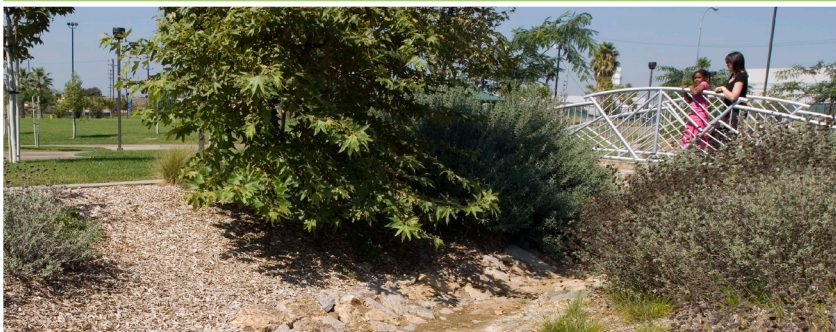
Figure 3 - 55: A pedestrian bridge extends over a dry creek bed, which collects storm water and filters it back into the LA River.
