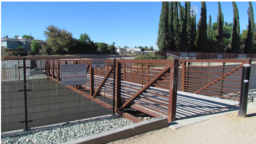
Figure 5 – 42: Browns Canyon Wash pedestrian bridge is a simple steel structure with a concrete platform that does not accommodate maintenance vehicles. (Location: Canoga Park).
