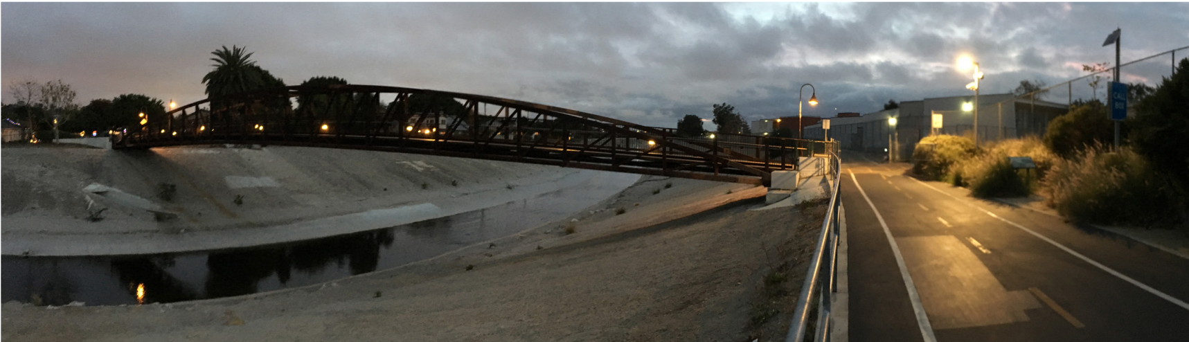
Figure 5 – 36: Ballona Creek pedestrian bridge at Westwood Boulevard. It is a through truss design that is wide and has lighting. (Location: Culver City).
