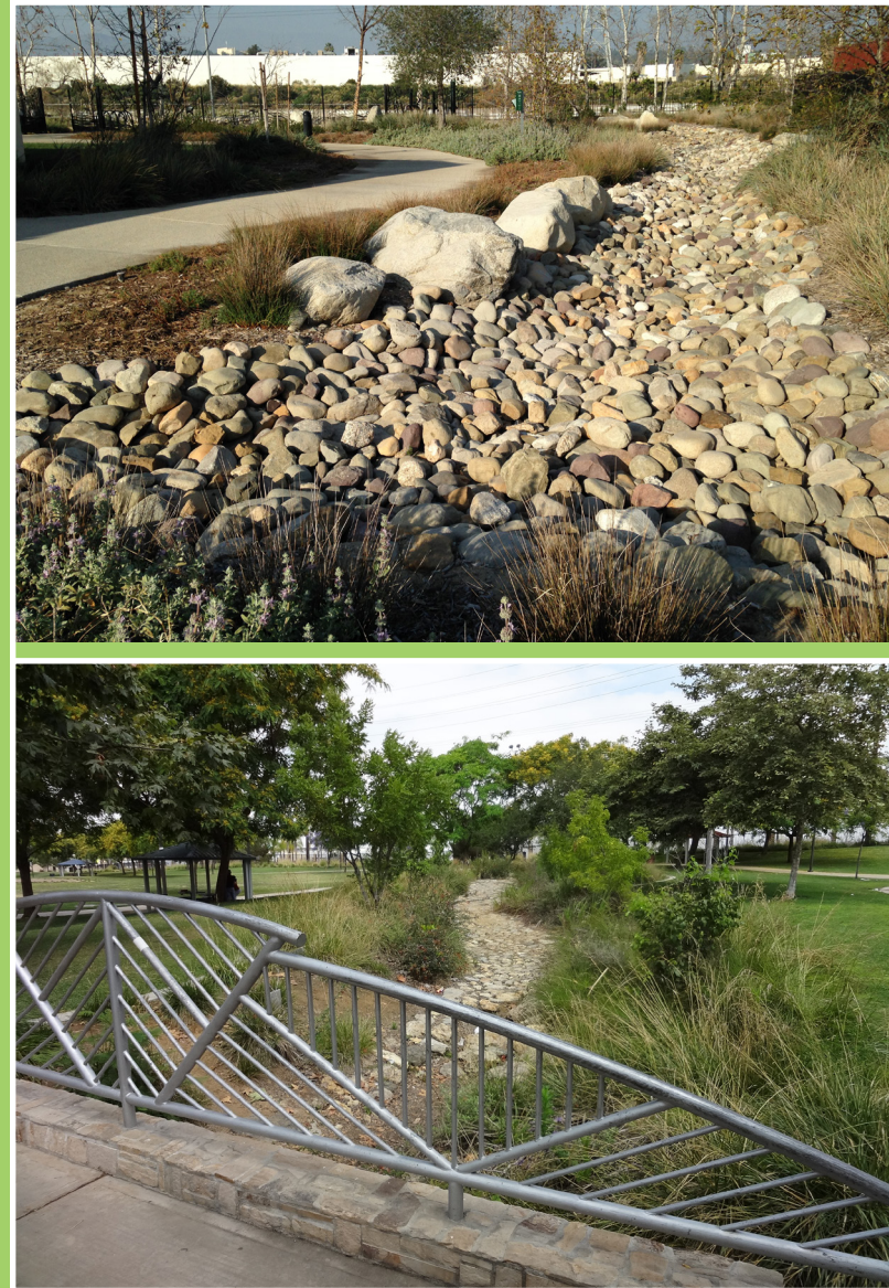
Figure 3 - 68: Example of a bioswale to capture, clean, and replenish stormwater above the LA River.
