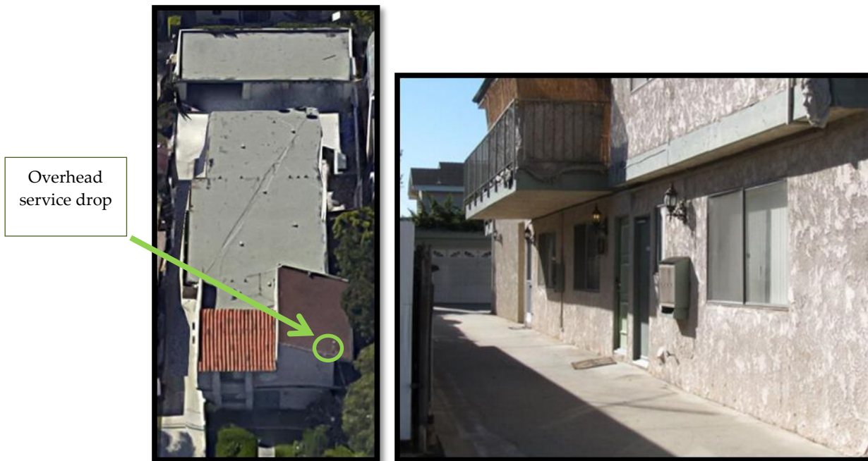
Photo Credit: Google Earth, On Target Electric
