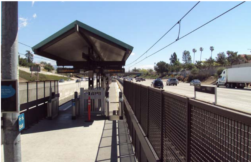
Figure 6: View of Canopy at Lake Station
