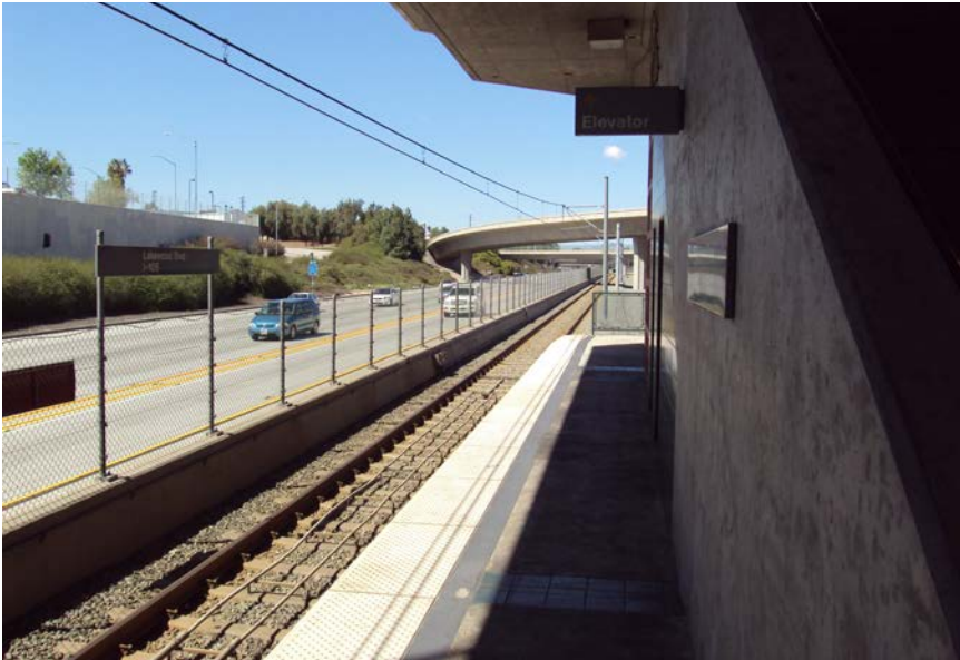
Figure 5: Wall Formed by Stairway at Lakewood Station
