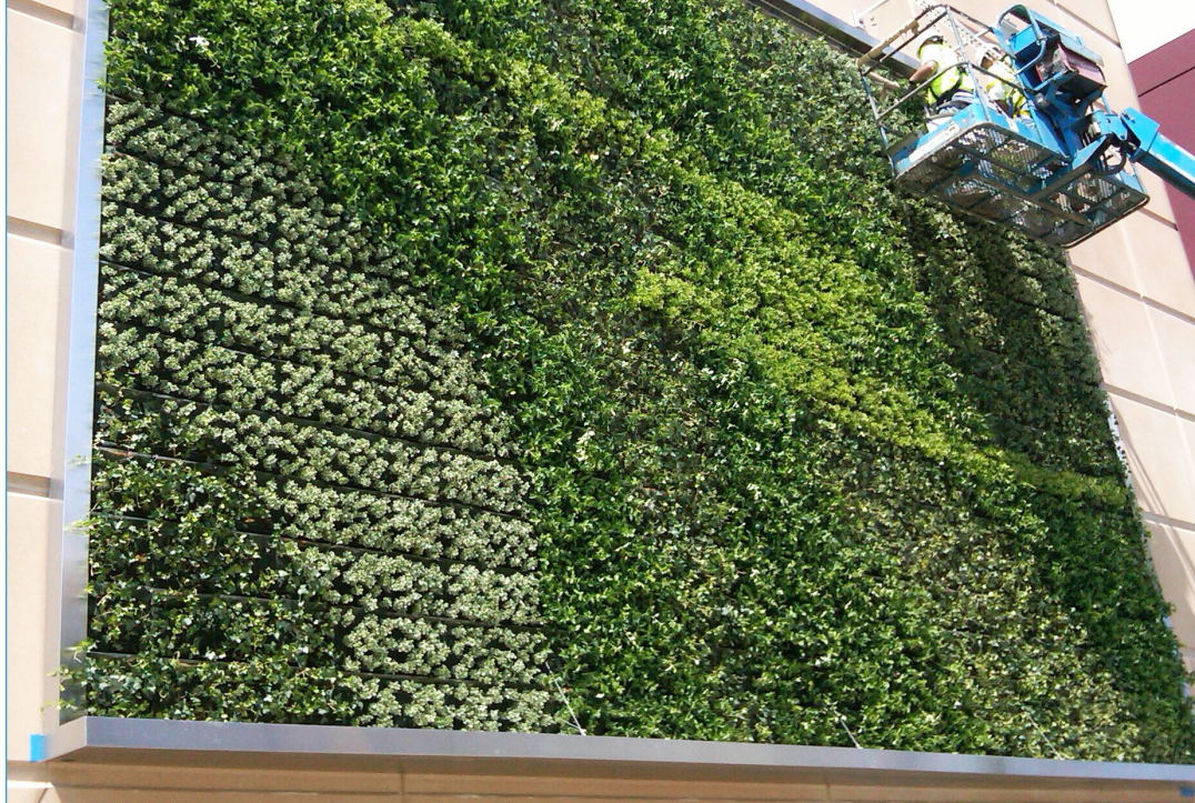
Figure 4:14: Green walls may be appropriate where vandalism deterrence is needed, but may require higher maintenance.
