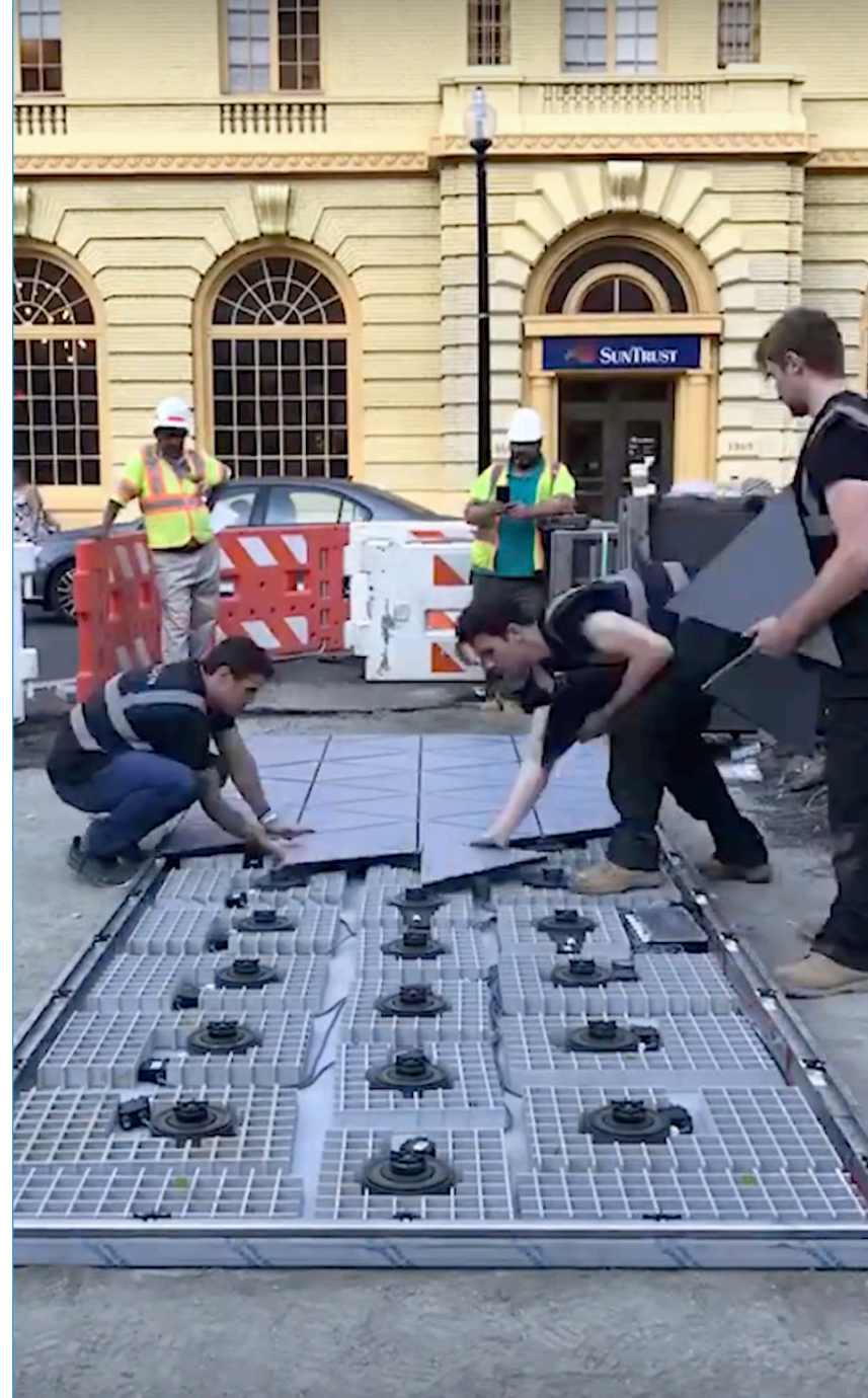
Figure 7.10: Piezoelectric tile is installed in Dupont Circle in Washington, D.C.
