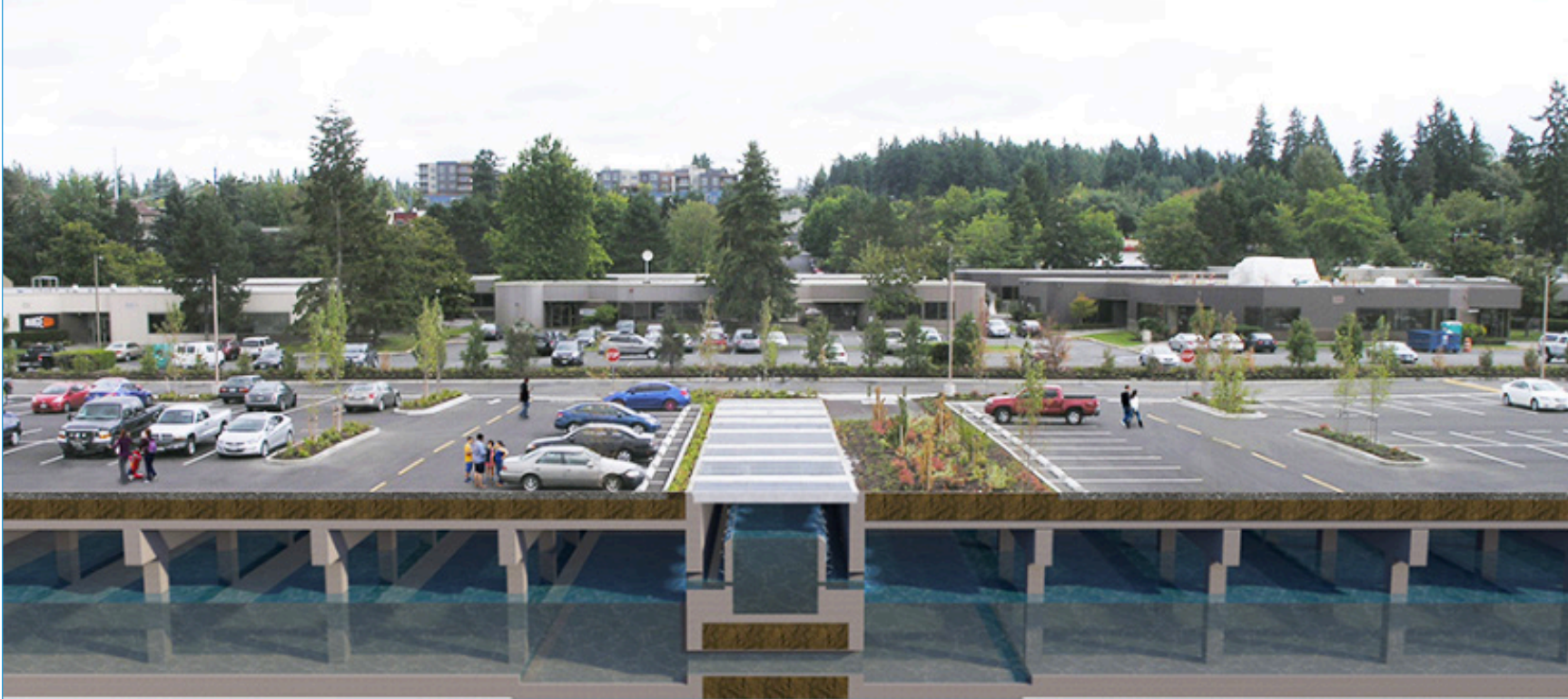
Figure 6.5: A rendering of the underground stormwater detention basin in Redmond, Washington, completed in 2015. It can hold 6.6 million gallons of stormwater. 12 At the time of construction, the surface was used for parking but there are plans to construct a park on its surface.
