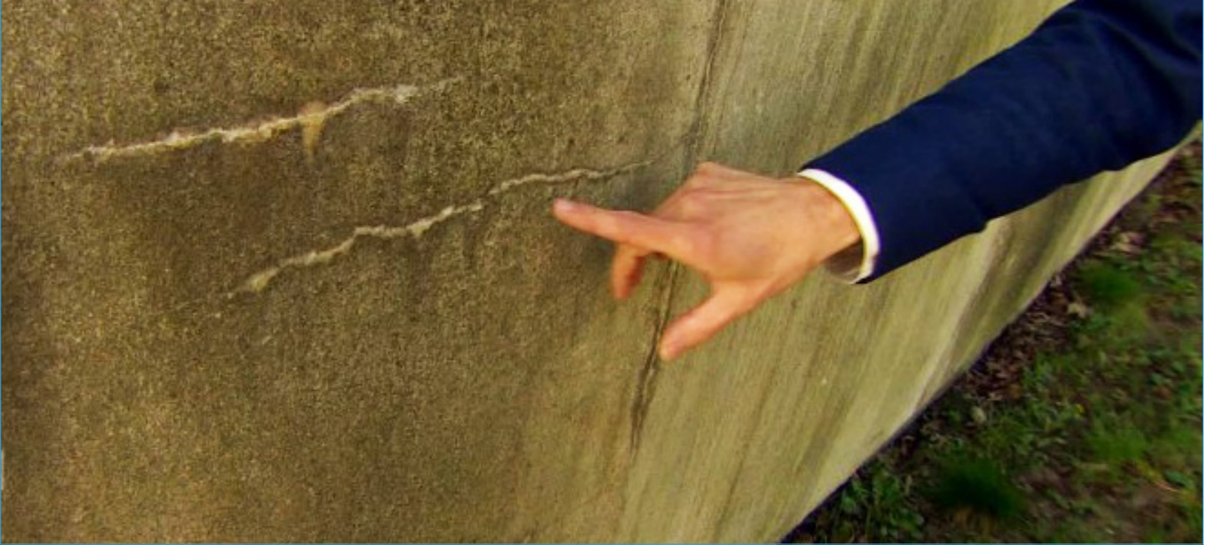
Figure 7.12: In bioconcrete, bacteria are activated and then germinate and multiply to form limestone in the “self-healing” process, leaving a mark.
