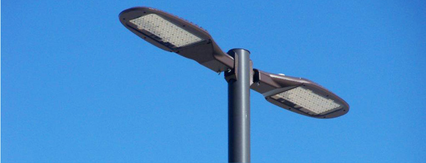
Figure 10.12: Light shields such as the flat version above focus the illumination, thus reducing light pollution and glare that can irritate the eyes.
