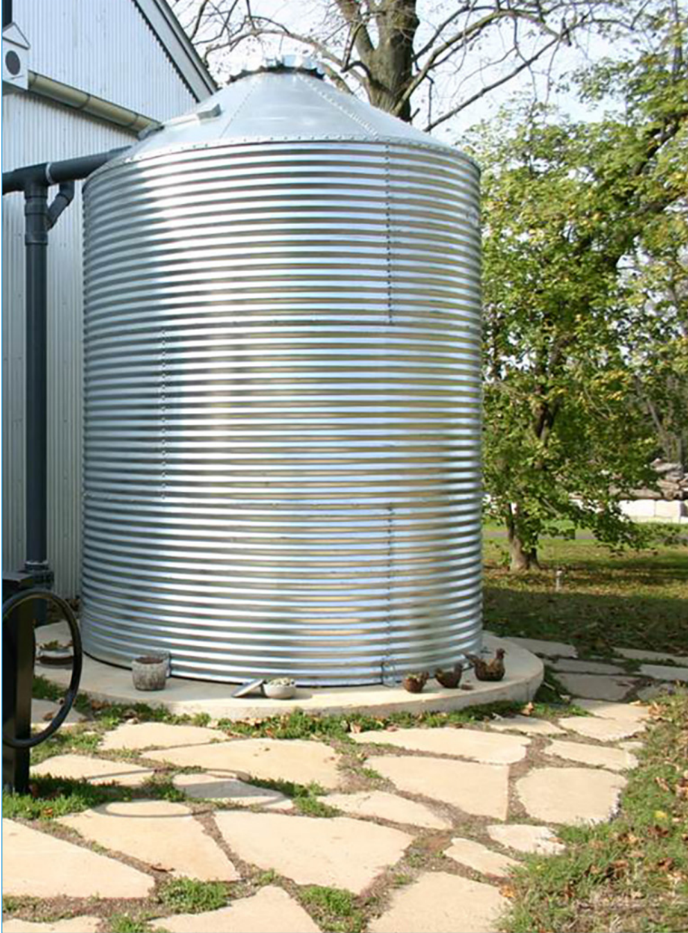
Figure 6.14: Rainwater harvesting into cisterns such as the one above can help reduce flood risk, alleviate drought, and enable park irrigation plans to adapt to changing climate.
