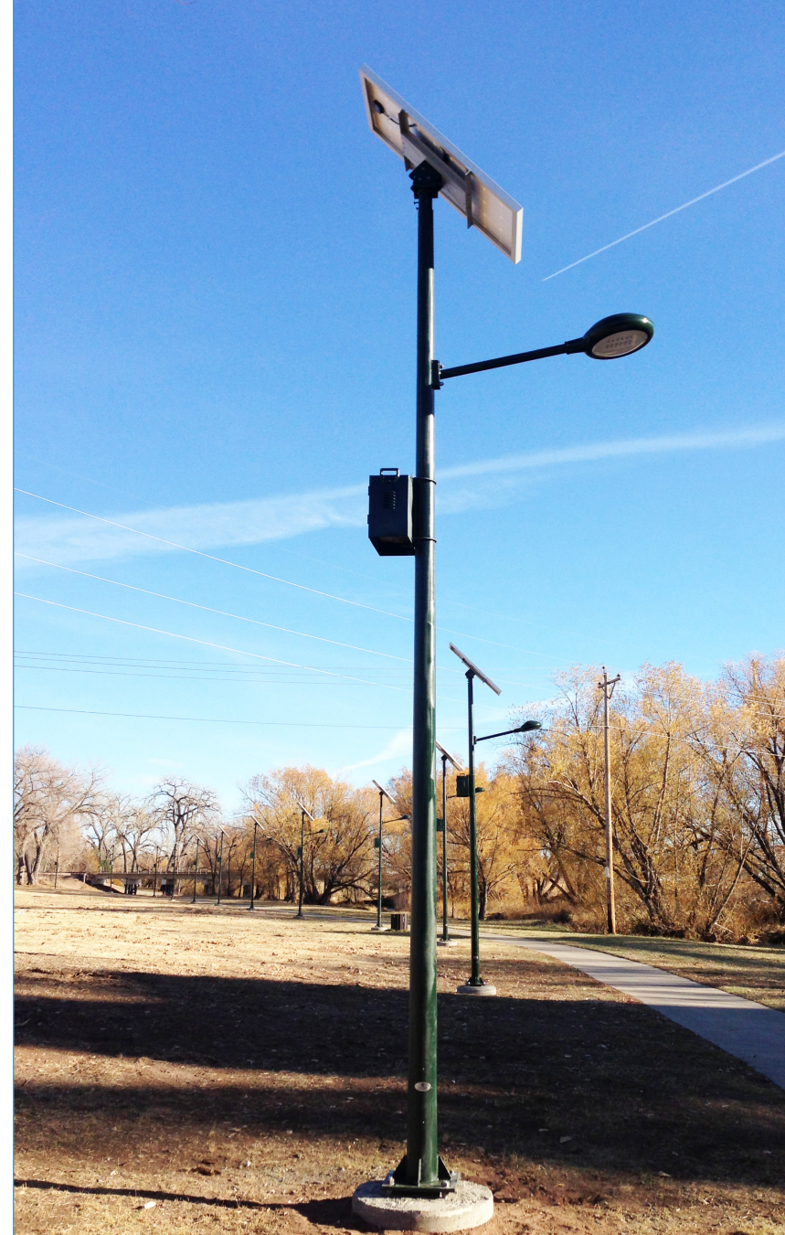
Figure 10.8: Off-grid light fixtures, powered by renewables, enhance park safety because they could operate during a local power grid outage.
