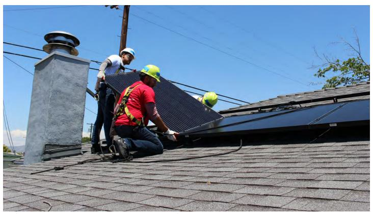
Rooftop solar PV panels installed by GRID Alternatives staff and trainees in Los Angeles. Photo credit: GRID Alternatives
