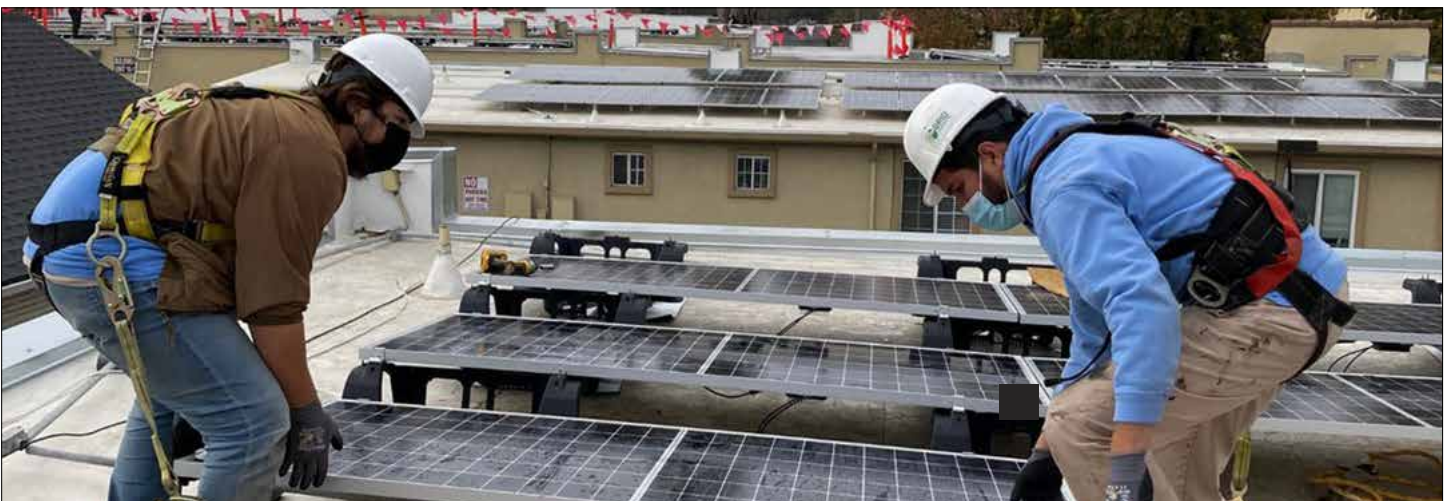
Solar installers from GRID Alternatives laying down PV modules at Casa de Oasis. Photo credit: GRID Alternatives
