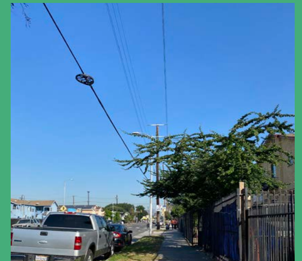
Figure 4. Overhead power lines
