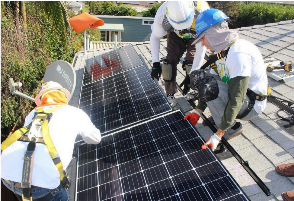
A GRID Alternatives team installs solar panels on a rooftop in Pacoima. Photo courtesy of GRID Alternatives
