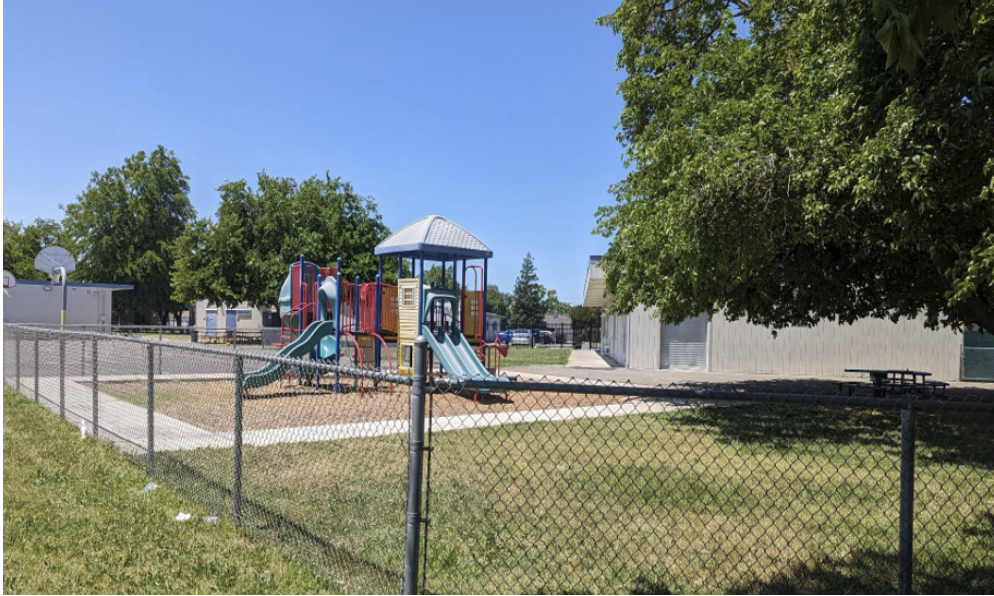
C. Portable classrooms surrounding an outdoor playground area in the Early Childhood Education Center at Parkway Elementary School in Sacramento City Unified School District (SCUSD), California. Source: Natalie van Doorn (2024)
