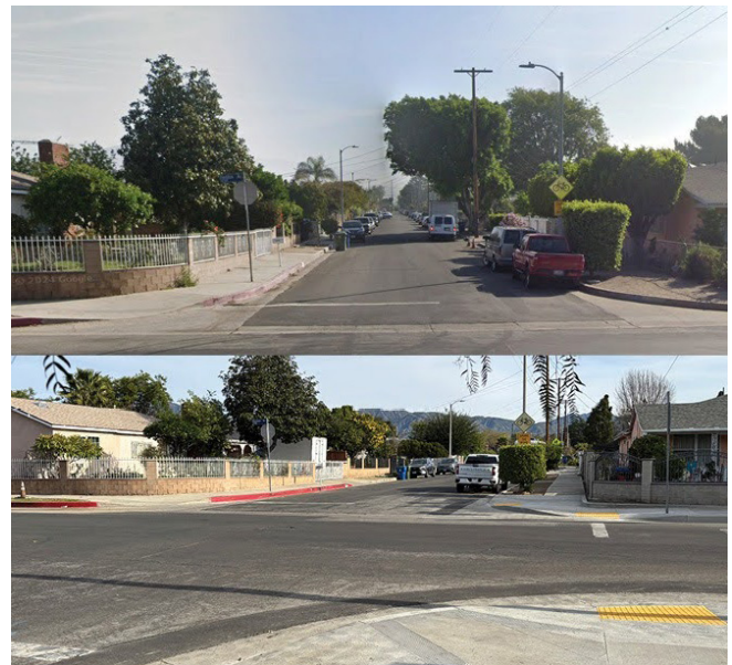
Haddon Avenue and Weidner Street in January 2015 (top). Same street in January 2026 after a sidewalk pavement, cut curbs, and improved signage were installed (bottom). Photo credit: Google Maps (top) & UCLA Luskin Center for Innovation (bottom)
