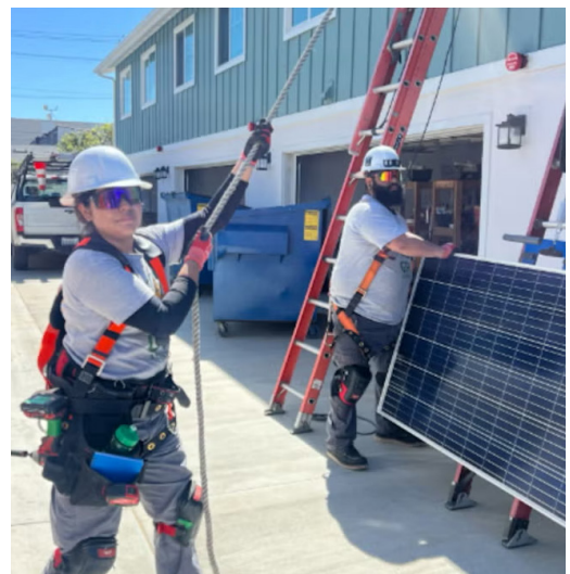
Angeles Martinez works on a solar installation during her training hours. Credit: GRID Alternatives Greater LA
